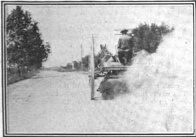
Before oiling the course it is thoroughly gone over with sweepers
